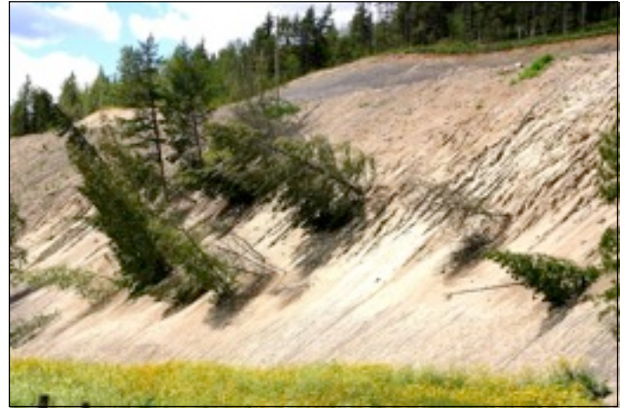
7.149 A landslide in the Rocky Mountains of Canada, near Jasper.
