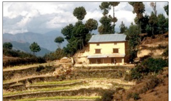
7.3 A typical house in Nepal, showing adaptation to the alpine climate. In Nepal, the houses are made from thick mud brick (adobe), which is an excellent insulator, and have small windows to contain heat loss. They are built on northern slopes to allow heating by the sun's rays.
