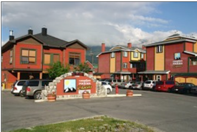
7.155 Substantial infrastructure supports tourism in alpine areas these days. These accommodation chalets are in the Canadian town of Jasper.
