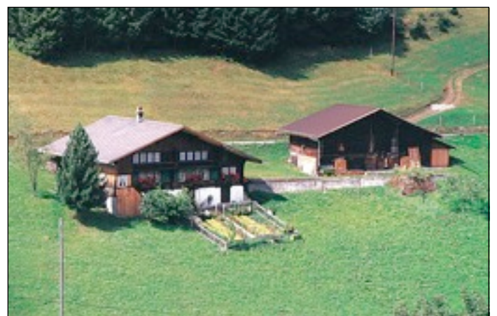
7.4 In Switzerland, many houses are made from thick timber (a good insulator) and the roofs have spikes to reduce the risk of avalanches of snow from the roof.
