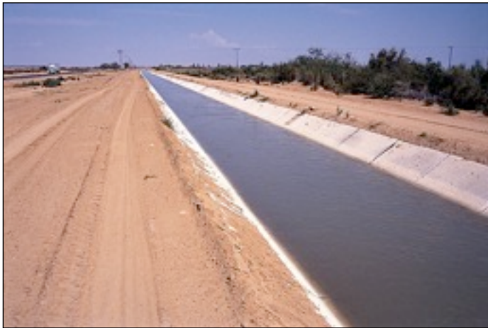
7.104 An irrigation canal bringing water from the Colorado River to southern California. There is considerable loss of water due to seepage and evaporation.
