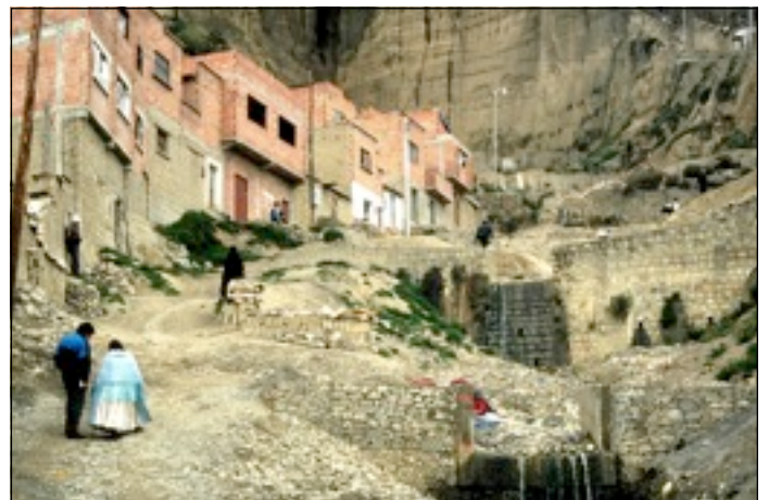
7.81 A poorer residential area of La Paz, situated on the upper edges of the canyon.
