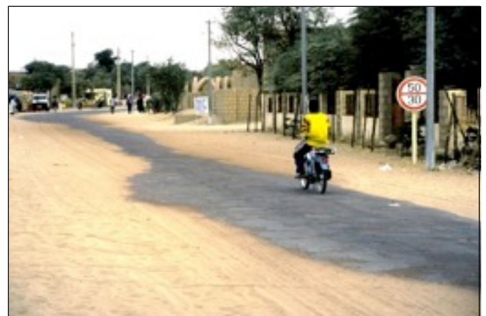
7.100 Although it is the largest town in northern Mali, Timbuktu has just one sealed road. Like Timbuktu itself, the road is becoming buried in sands that blow in from the surrounding Sahara Desert.
