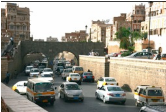
7.144 The ephemeral stream known as Wadi as Sa'ilah, in Sana'a, has been converted into a canal which is used as a roadway when the stream is not flowing.
